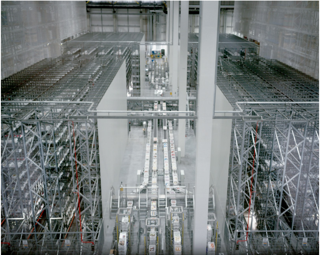
Logistiikkakeskus (Workers have left the factory), 2021
